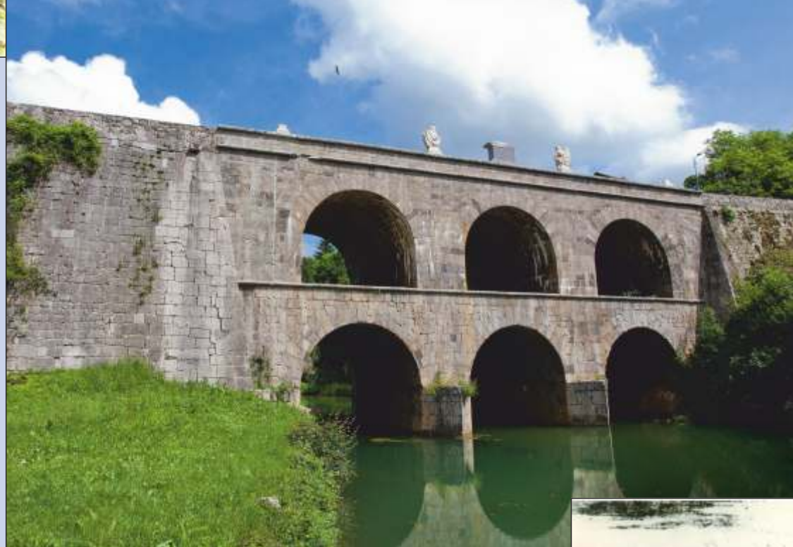
Tounjski most Tounj bridge
